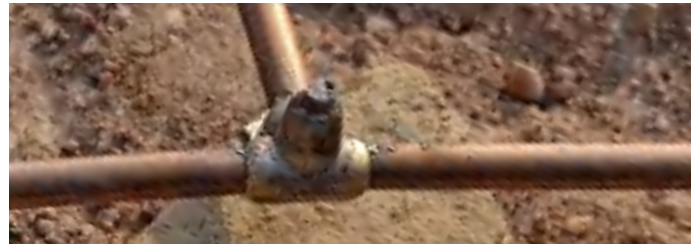
TA nVent ERICO Cadweld connection
