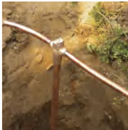
GT Cadweld connection
